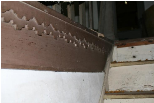
Figure 132: Alfred Jackson Mizelle House, enclosed stair with scalloped trim.
