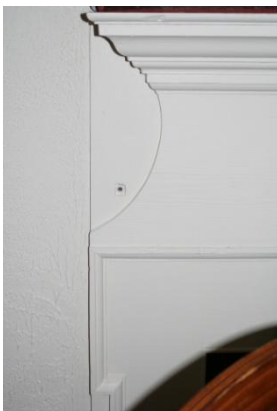
Figure 27: Samuel and Sallie Adams House, ca. 1908, detail of mantel believed to be from earlier ca. 1800 Nicholls-Webb House formerly on site. Note crossette.
