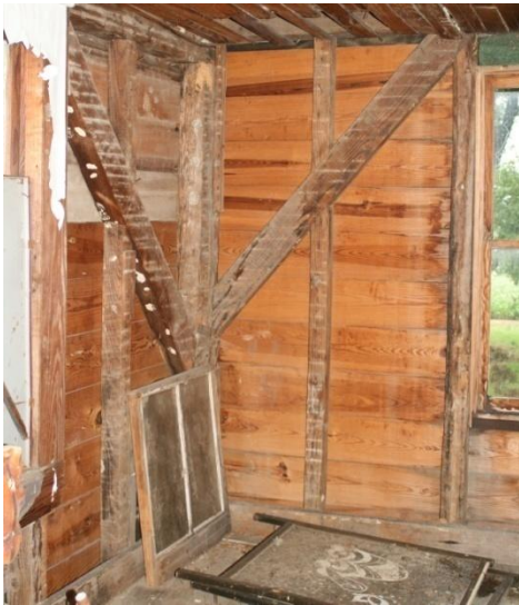
Figure 6: Ward House, ca. 1850-1860, floor plate and ends of floor joists, studs (interrupted by new window) and down brace.
