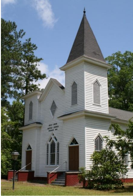
Figure 200: Holly Grove Baptist Church, 1860, remodeled 1911-1912.
