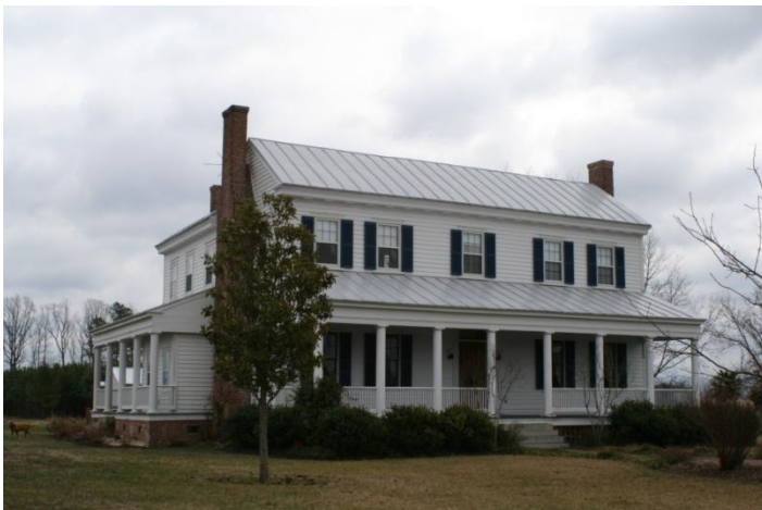
Figure 60: Ashland. Note two-story ell extending to rear.
