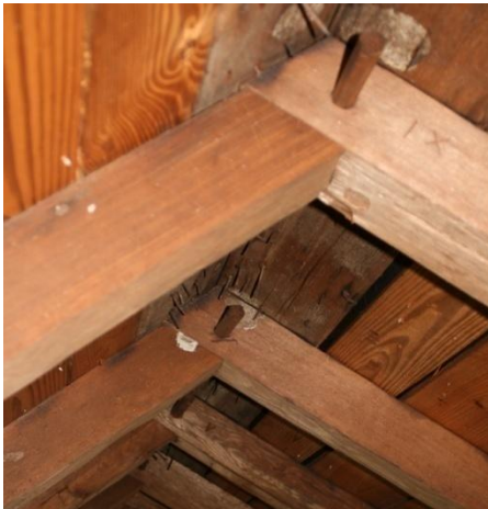
Figure 8: Bond-Haste House, ca. 1800-1810, finely squared, numbered, and pegged mortise and tenon rafters.
