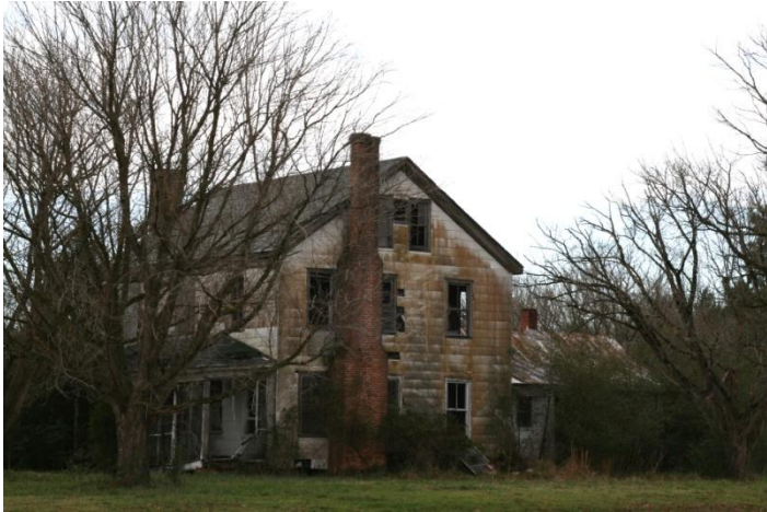
Figure 29: Asa Phelps House. Note the double shouldered exterior end chimneys and double pile form.
