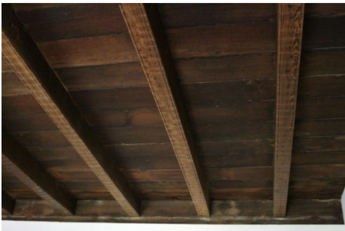
Figure 18: R. A. Cowan House, beaded ceiling joists.
