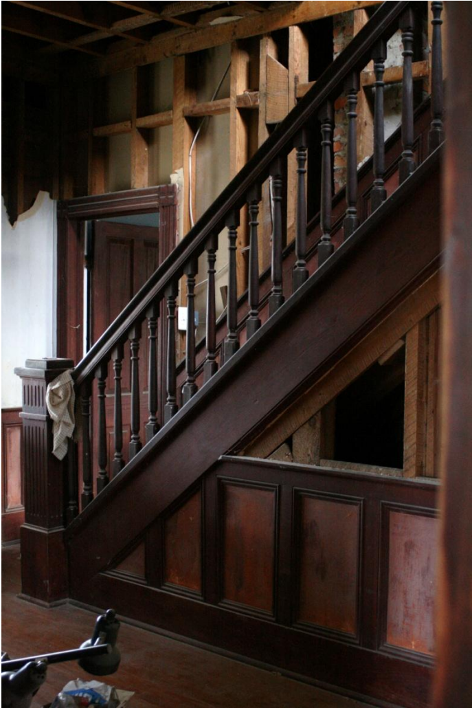
Figure 165: Eastbrook, center hall showing two-by-four framing and Victorian staircase.
