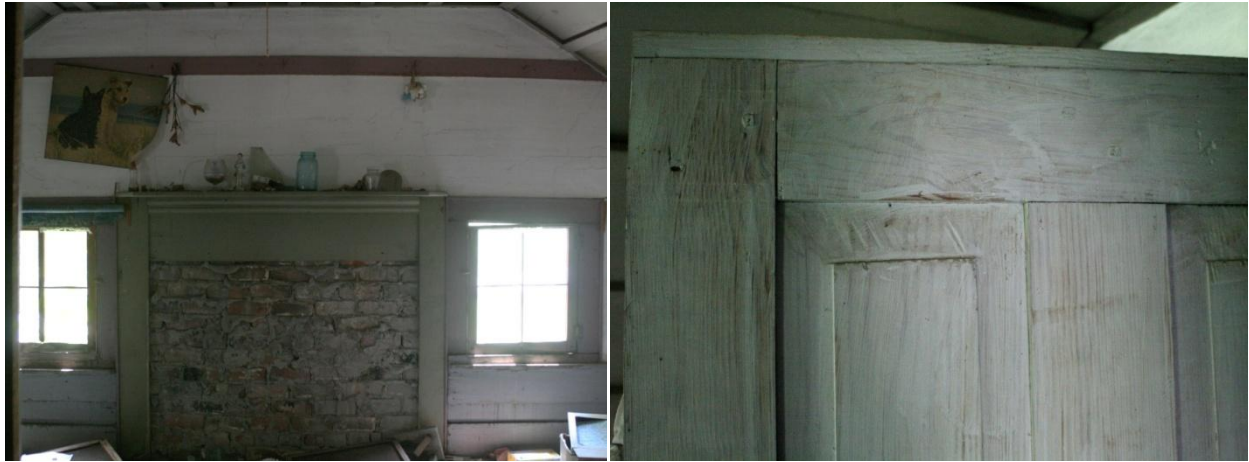
Figure 130: Alfred Jackson Mizelle House, second floor chamber. Figure 131: Hand-planed, pegged door.
