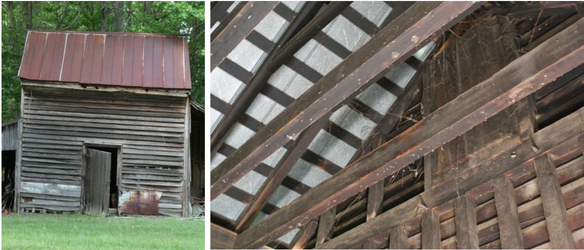
Figure 88 and Figure 89: Bond-Haste House smokehouse, ca. 1810. Note close spacing of studding.
