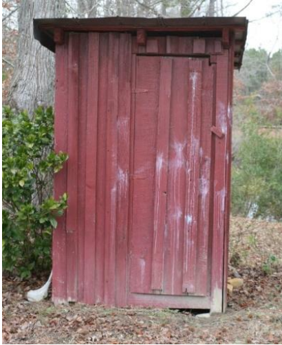
Figure 197: Frank Phelps House privy.
