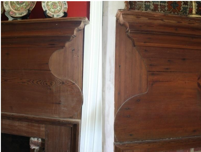
Figure 23: Garret-White House, mantel frieze and shelf profiles side by side.
