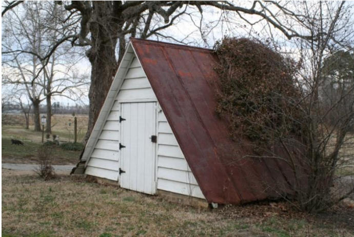
Figure 95 Figure 96: Mill Landing icehouse and view looking down into interior.
