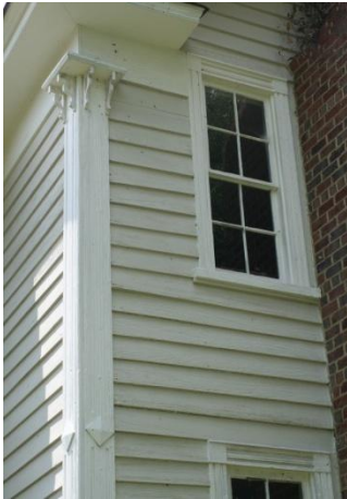
Figure 115: Abram Burden House, 1871, corner pilaster detail.
