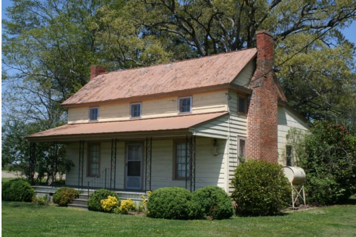
Figure 127: Annie Baker House, ca. 1875. Story-and-a-half with over porch windows and side chimneys.
