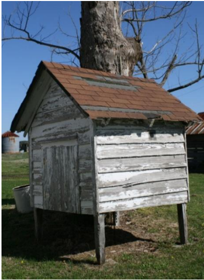
Figure 149: Lane-Forehand stilted dairy.
