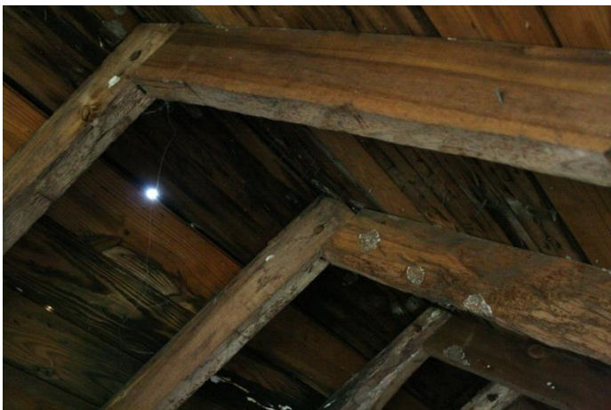
Figure 9: Asa Phelps House, ca. 1810-1815, roughly sawn and hewn, numbered, and pegged mortise and tenon rafters. Note waney edges and varying sizes of rafters.
