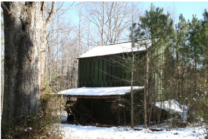
Figure 187: Clarence Hoggard tobacco barn, with ridge vent and shelter over door.
