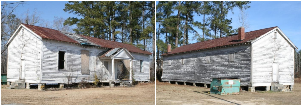
Figure 220 and Figure 221: Ashland School, ca. 1920-1930.
