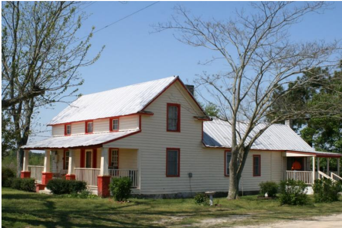
Figure 126: Mitchell House II, ca. 1890-1910. Story-and-a-jump with front over porch windows and rear chimneys.
