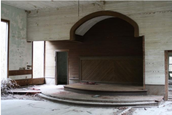
Figure 153: White Oak Methodist Church, 1914 interior remodeling.
