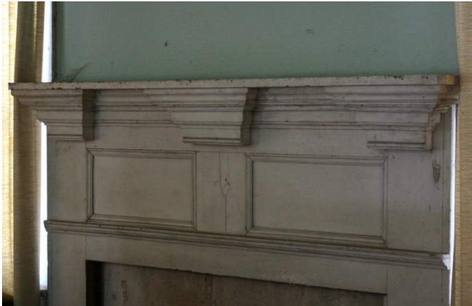
Figure 52: Starkey Evans House, hall mantel.
