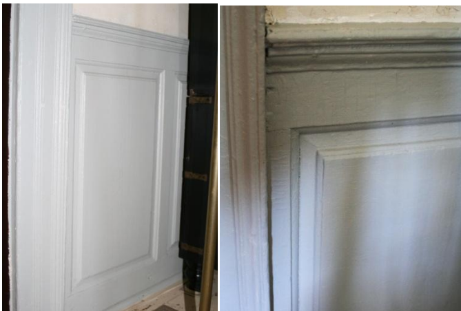
Figure 24: Garret-White House, double lip raised panel wainscoting.
