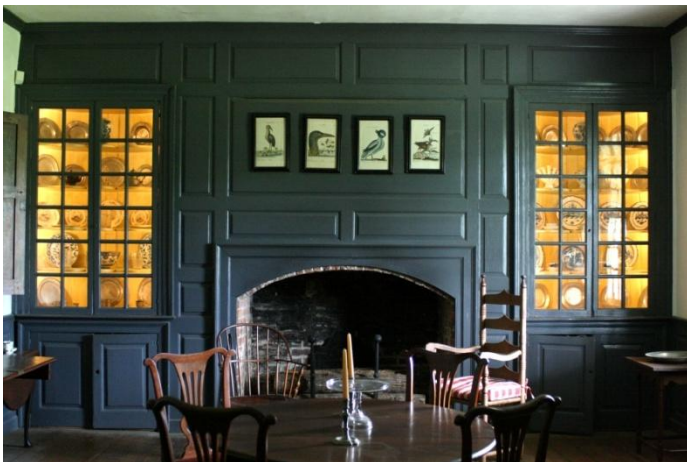
Figure 15: King-Bazemore House hall, paneled end wall with cupboards.
