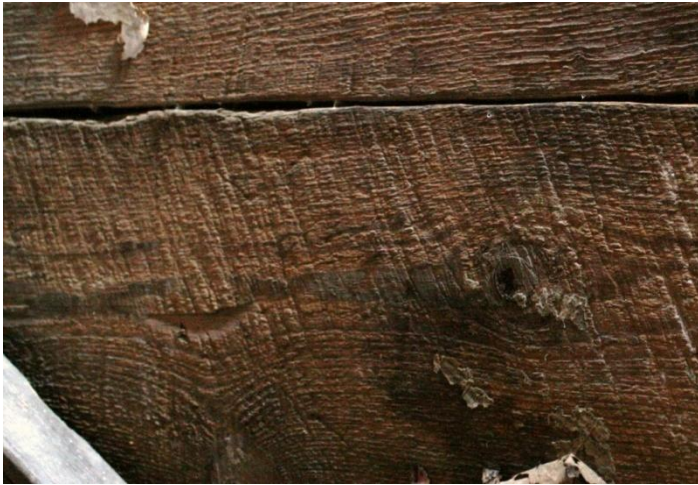
Figure 11: Seay Building, interior detail of corner dovetail with incised numeral.
