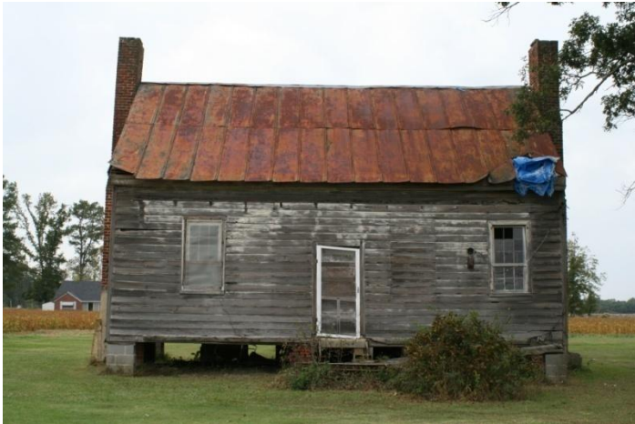
Figure 47: Carter House, ca. 1810-1830, original rear, now front elevation.
