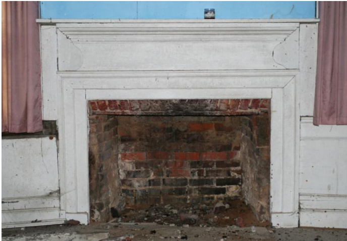
Figure 25: Mitchell House, ca. 1805-1815 and ca. 1850-1860, mantel of older section. Note that ogee curves of frieze on each side do not match each other exactly.
