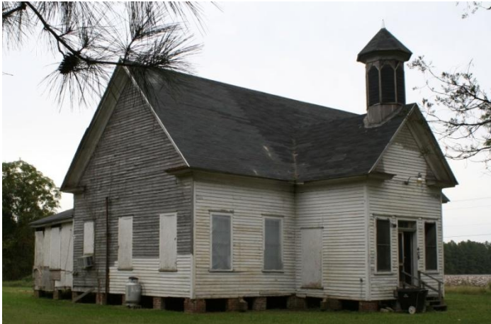
Figure 211: Kelford School, ca. 1910.
