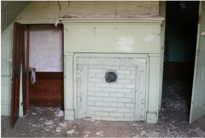
Figure 46: Bazemore House, second floor chamber.
