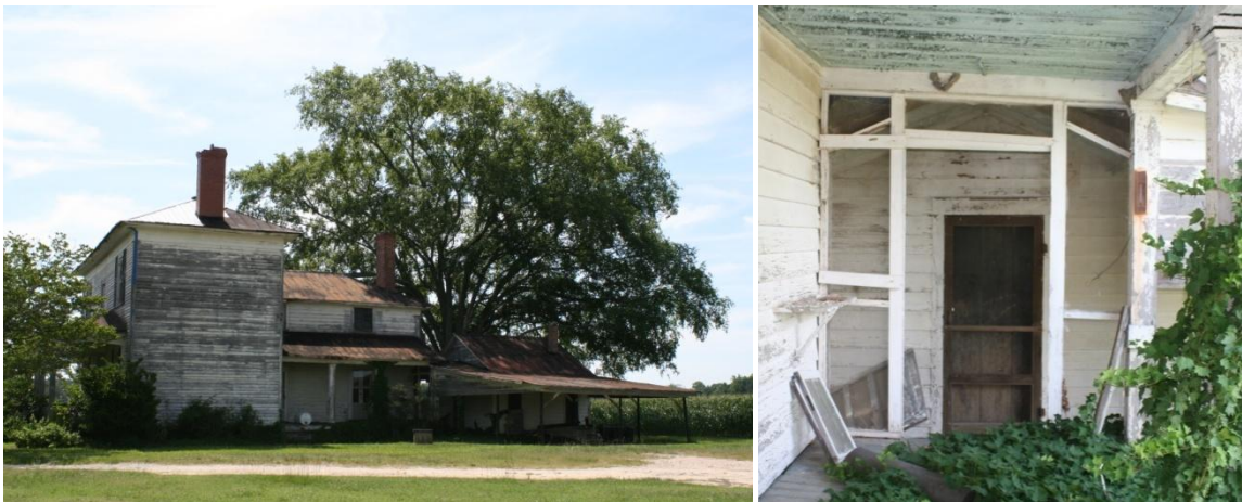
Figure 82 and Figure 83: King-Grant-Alston House, ca. 1850-1860 with kitchen to rear (car shelter is later addition). View of kitchen door from side porch of dining room (small gable roof between porch and kitchen is a later addition).
