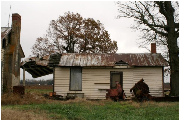
Figure 84: Cox House, ca. 1850-1860, kitchen with back of house to left.
