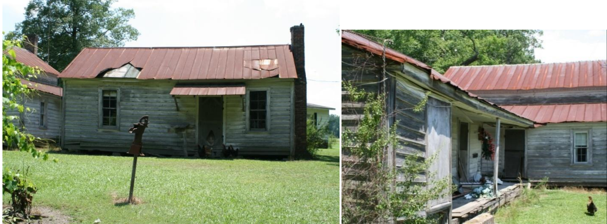
Figure 142: Alfred Jackson Mizelle House, ca. 1880-1900, side elevation of kitchen and dining building connected to house at left by short breezeway. Note pump in foreground. Figure 143: View of kitchen colonnade and breezeway from rear.
