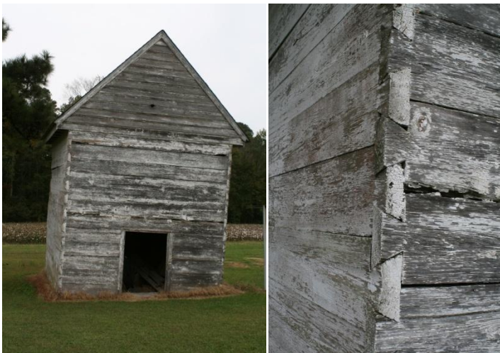
Figure 86 and Figure 87: Pineview, ca. 1840 smokehouse and detail of full dovetails.
