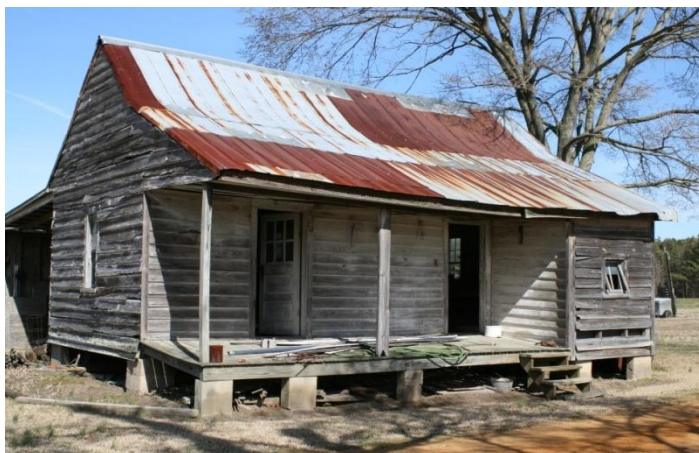
Figure 145: Thadeus A. Perry House, ca. 1870-1890, detached kitchen and dining building. (House has been moved away from building.)
