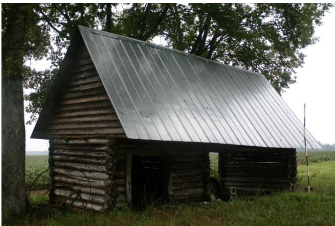
Figure 193: Castellow-Tarkington storage shelter, ca. 1935.
