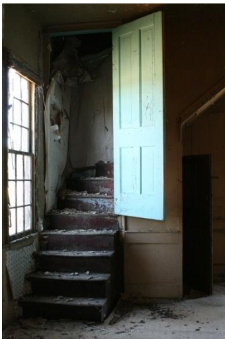
Figure 45: Bazemore House, partially enclosed winder stair.
