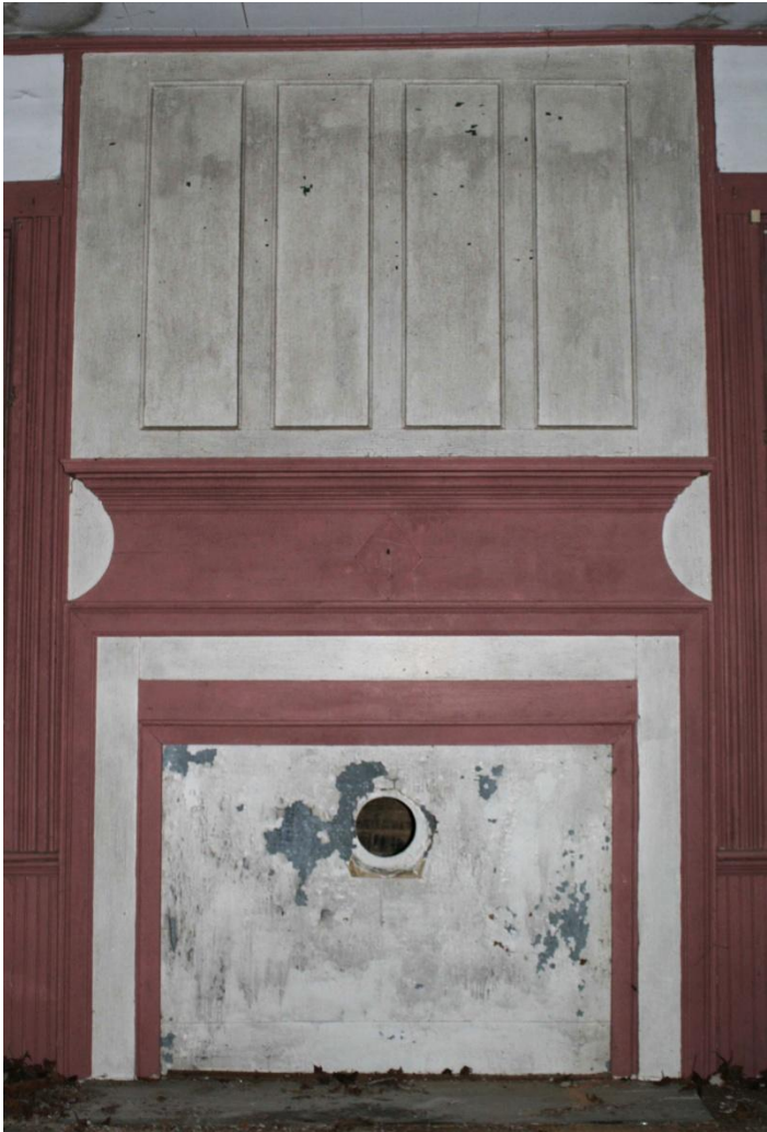
Figure 28: Asa Phelps House, ca. 1810-1815, fist floor Georgian-Federal mantel and overmantel.
