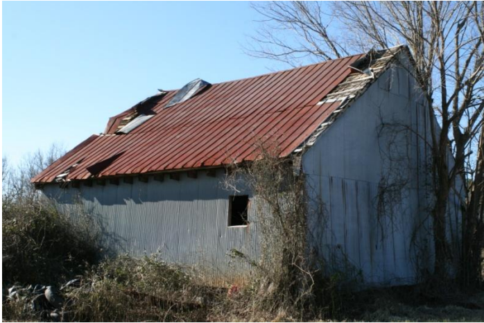
Figure 106: Mitchell House barn, ca. 1850-1860.
