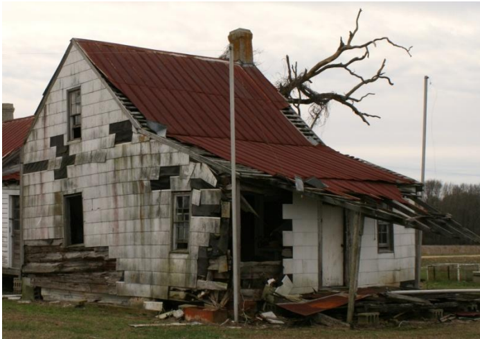
Figure 19: Seay Building, ca. 1780-1800.
