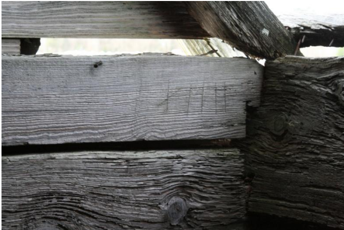
Figure 12: Bucklesberry smokehouse, dovetail detail.
