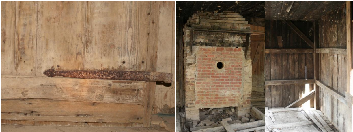
Figure 110: Jeremiah's House hook and eye hinge. Figure 111: Fireplace. Figure 112: Post and rail frame.
