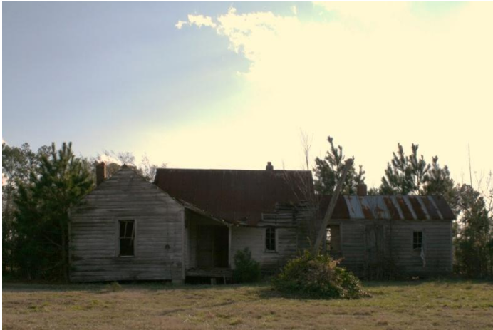
Figure 183: Willow Branch Farm, tenant house, ca. 1910-1920.
