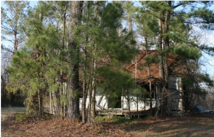
Figure 185: Willow Branch Farm, tenant house, ca. 1920-1930.
