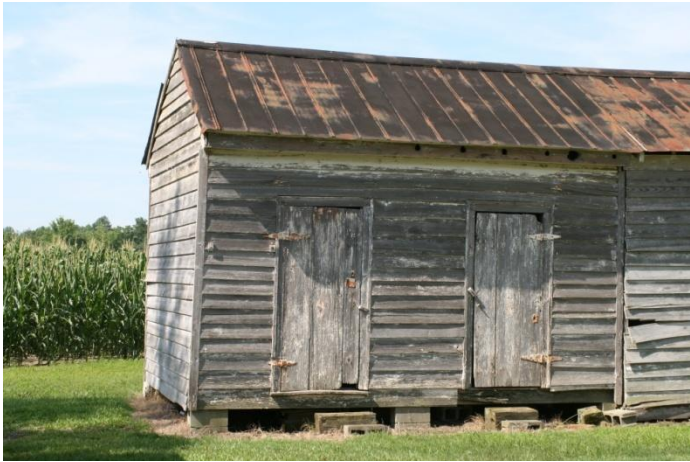
Figure 94: King-Grant-Alston House, ca. 1850-1860 outbuilding (section at right edge of photograph is later addition).
