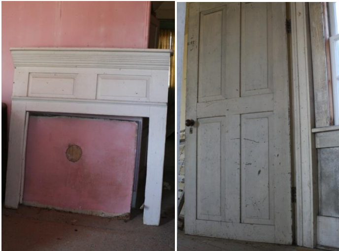
Figure 53: Starkey Evans House, raised panel mantel first floor and raise panel door second floor.
