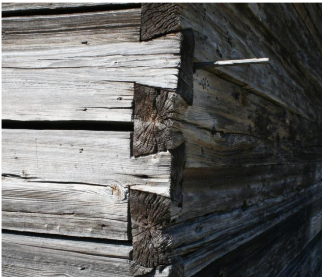
Figure 12: Bucklesberry smokehouse, dovetail detail.
