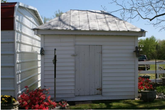
Figure 194: Miller-Brown generator house.
