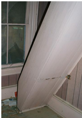
Figure 32: Asa Phelps House, stair to attic. The gentle undulations in the surface of the boards left by the hand plane are just visible.
