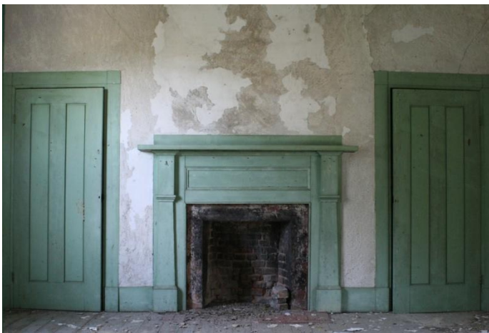
Figure 64: King-Grant-Alston House, second floor chamber.
