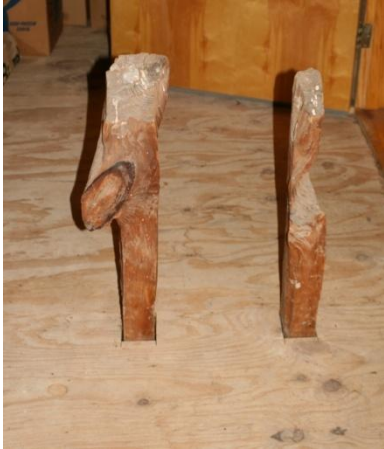
Figure 74: Liberty Hall, studs projecting into attic.
