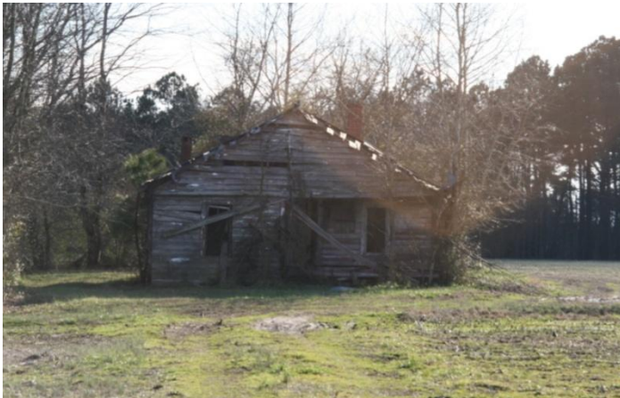
Figure 186: Willow Branch Farm, tenant house, ca. 1930-1940.
