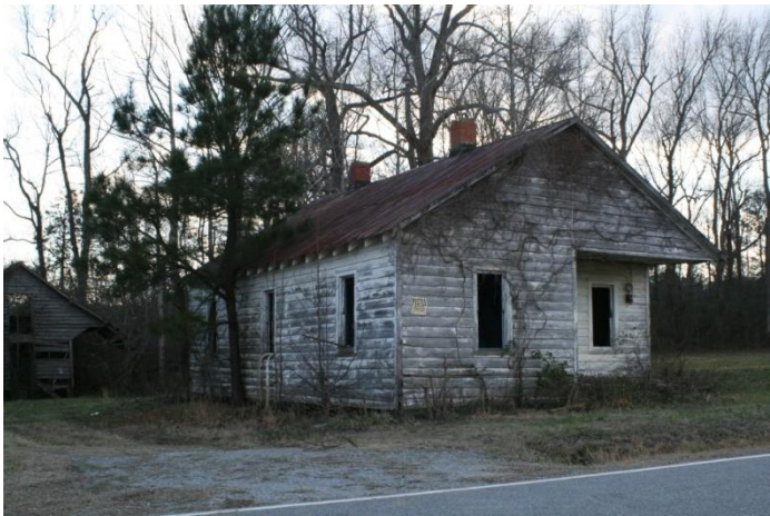
Figure 184: Willow Branch Farm, tenant house, ca. 1930-1940.
